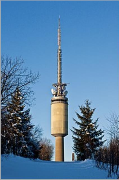
Tryvann Tower, February, 2010
